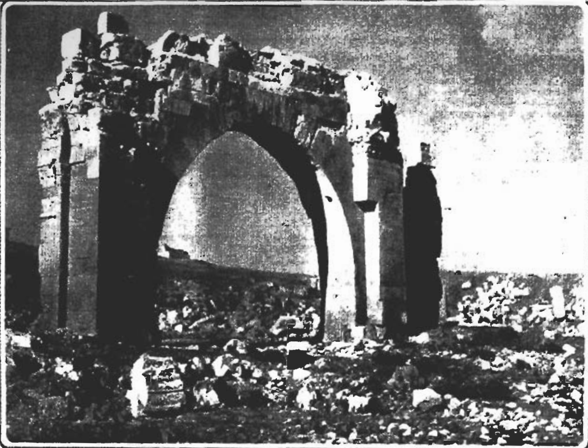
FIG. 4. THE GREAT ARCH OF THE COURT-FACÈDE OF THE MOSQUE SANCTUARY. THE ARCH SPAN IS 27 FT.
